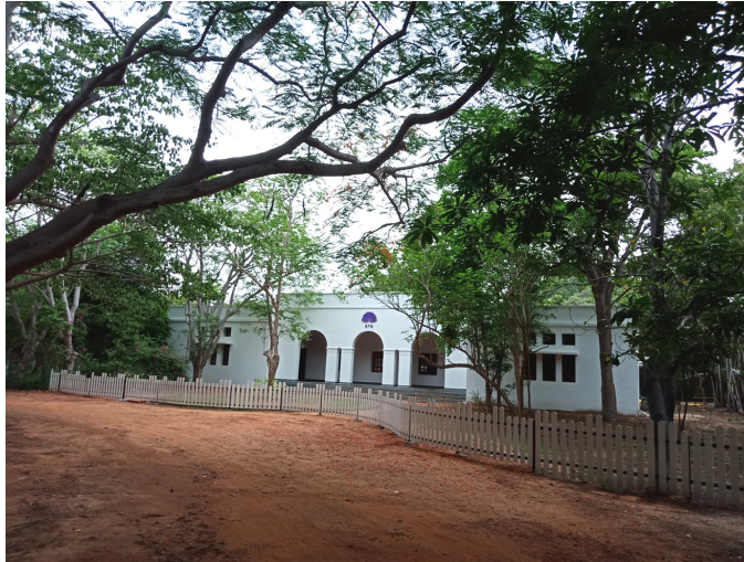
The newly renovated ATA building
